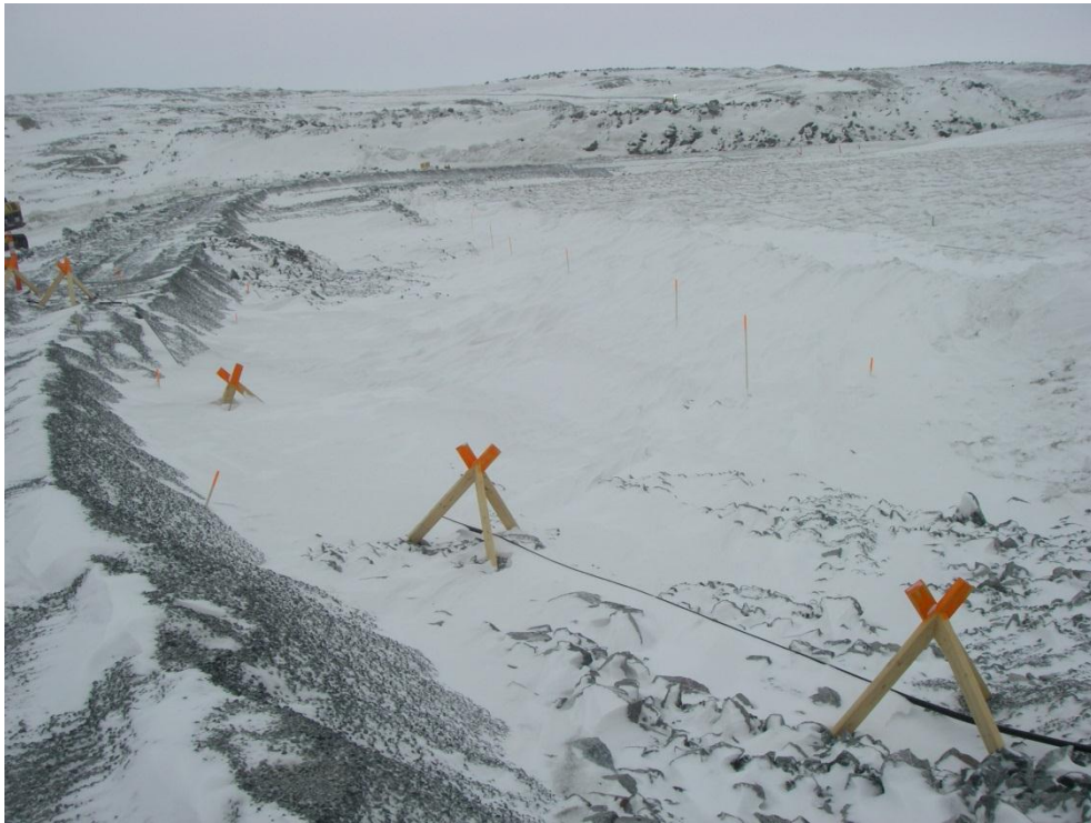
Photo 5: Diversion Berm – snow drifted in on the upstream side of the berm. Photo looking west from Sta. 0+150.
