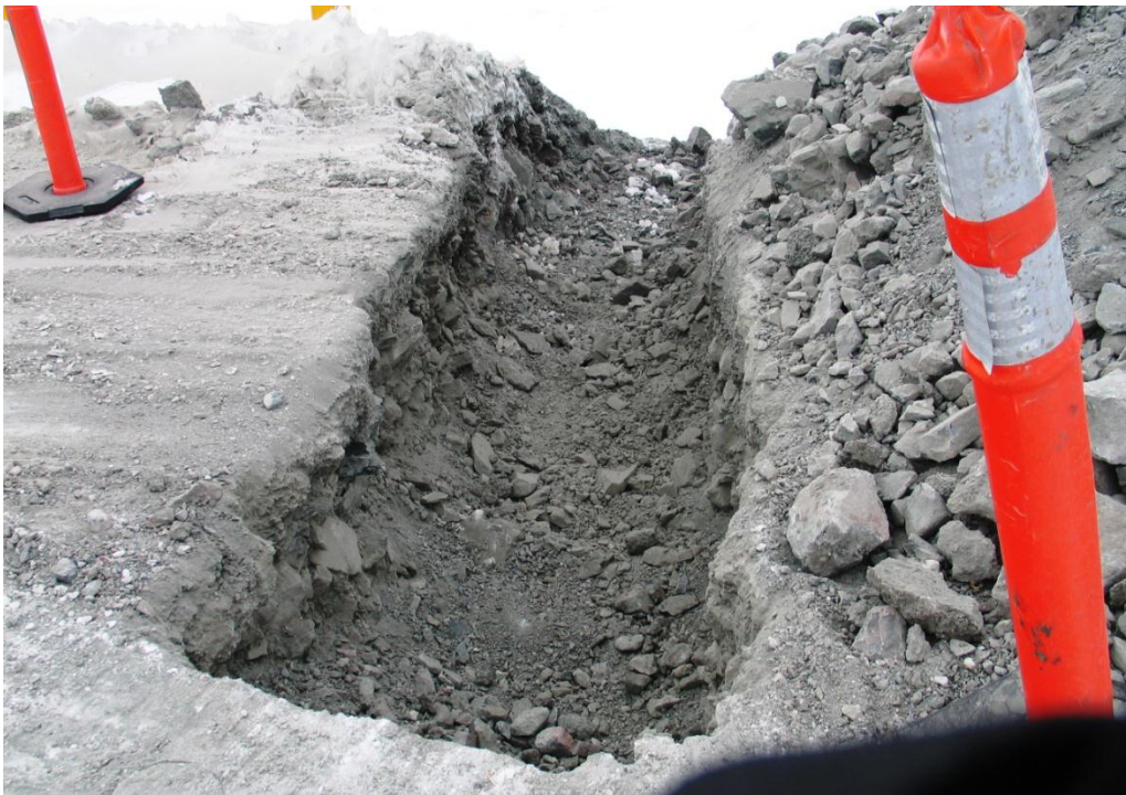
Photo 7: Excavation for thermistor cable installation at Bridge#4.
