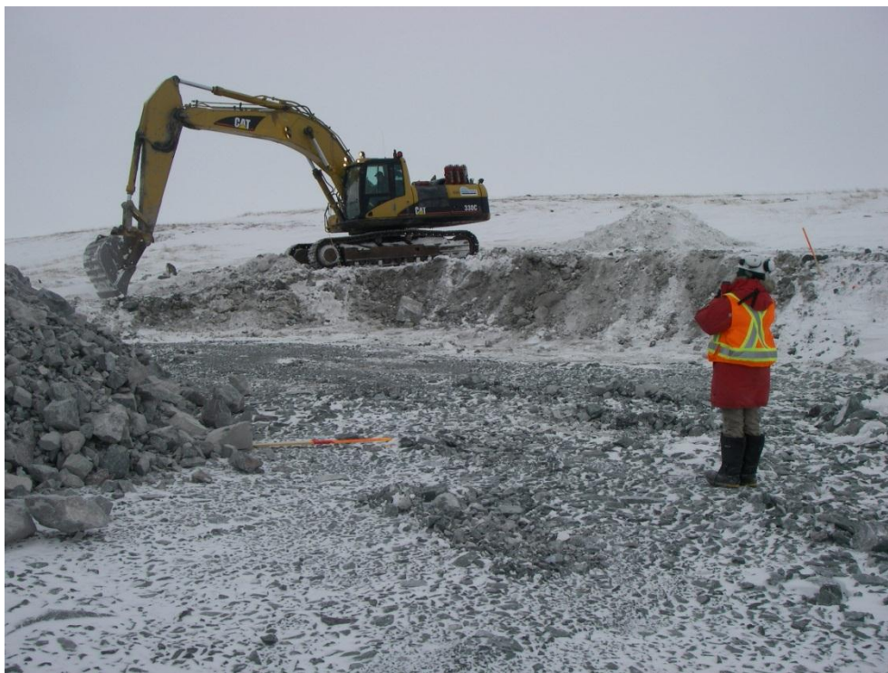
Photo 4: North Dam – clearing snow ahead of ROQ placement. Photo looking south from Sta. 0+30.
